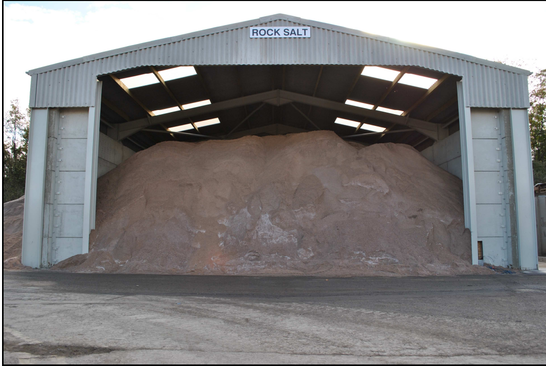
Salt barn Storage capacity 850t
